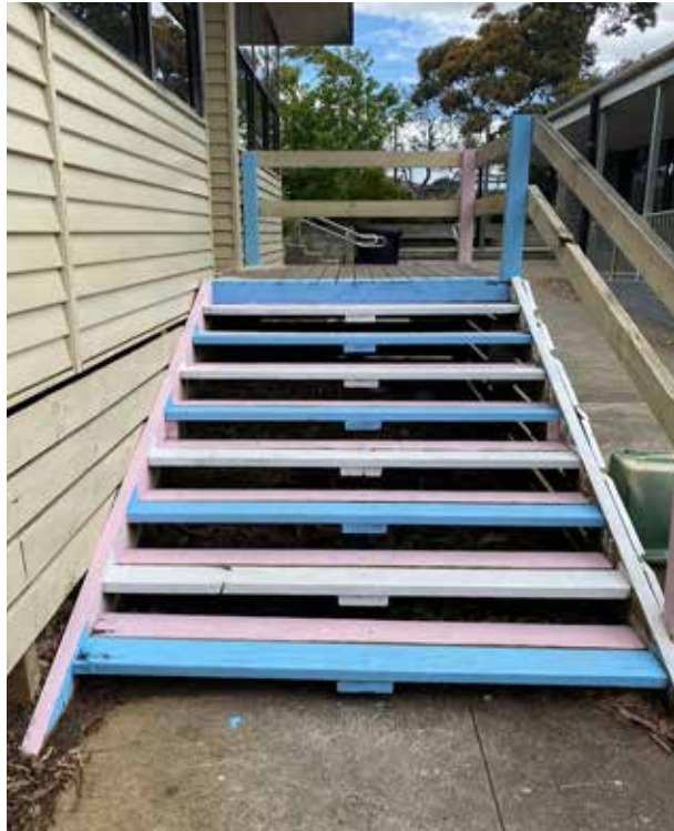
The newly painted steps to the Wellness Zone on the Junior Campus
